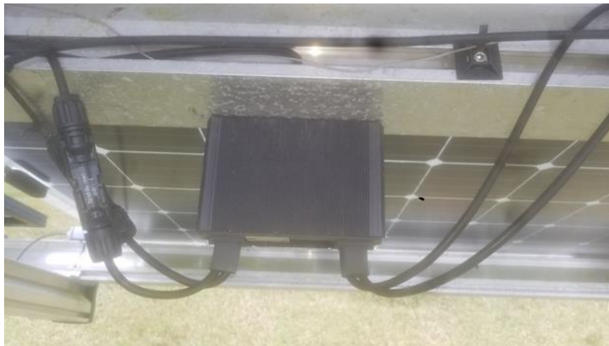
Figure 4.3: OUC's DC Optimizer Configuration by Maguire Mulligan.
