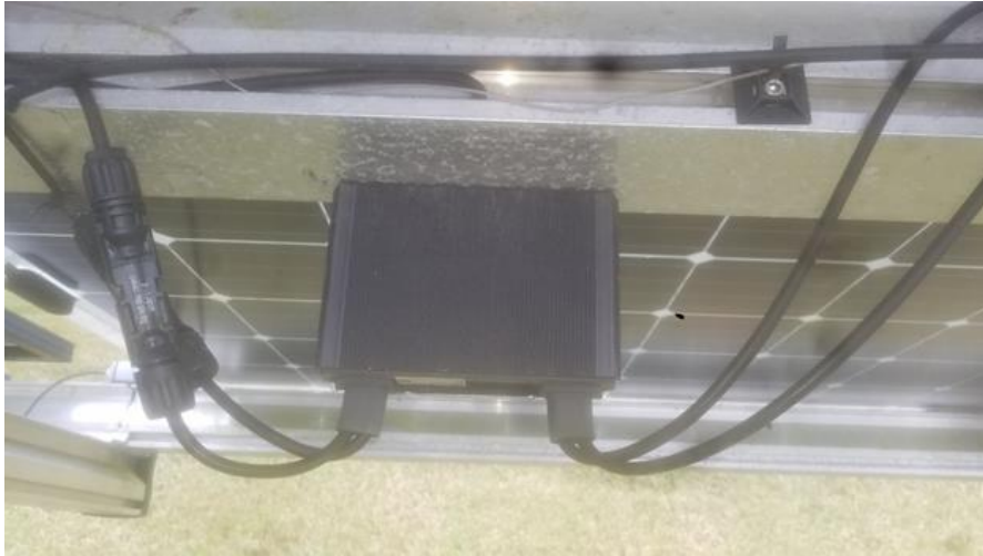
Figure 4.2. OUC's DC Optimizer Configuration
