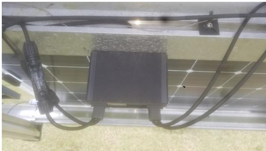
Figure 4.2. OUC's DC Optimizer Configuration
